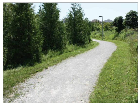
GRANULAR PAVING - LIMESTONE SCREENING
