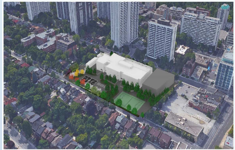
Land lease to City for new aquatic centre at Davisville JPS site
