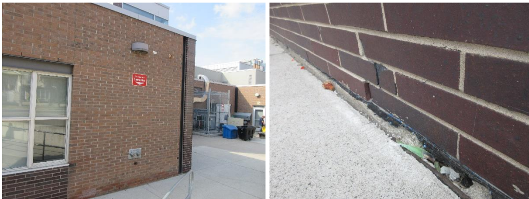
Brick conditions- deterioration/ damage at grade
