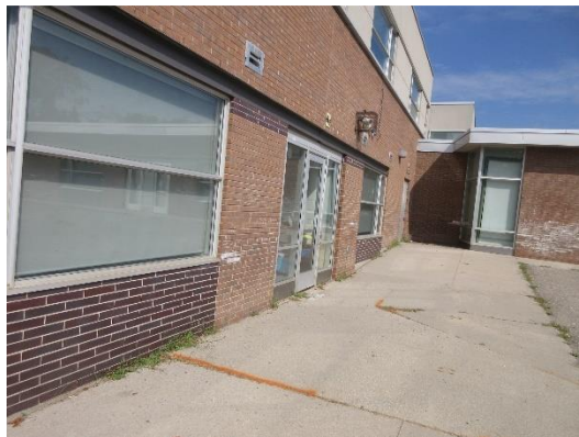
Staining/rust at grade- Aluminum doors & steel columns
