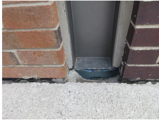
Concrete Walkways settled in a number of areas
