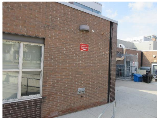
North Façade- Fire Department Connection
