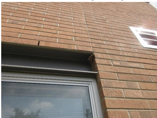
Exposed steel columns & Beams as window surrounds
