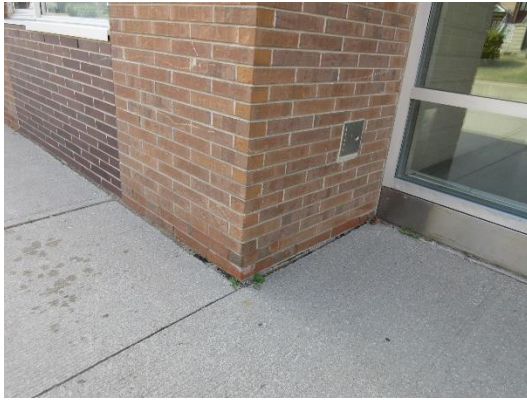
Concrete Walkways settled in a number of areas
