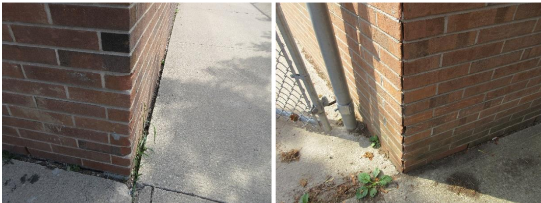
Brick conditions- chipping at corner joints
