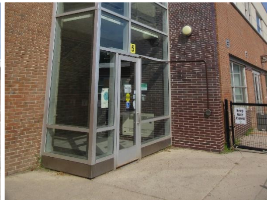
Staining/rust at grade- Aluminum doors & steel columns
