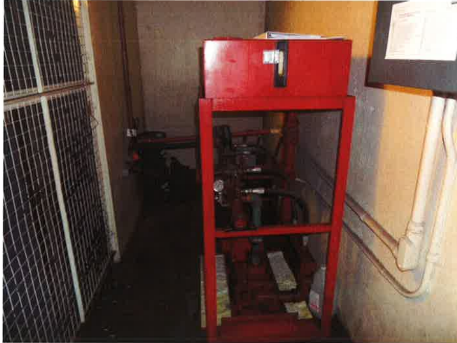
Photograph 5: View of the hydraulic cage for the elevator. Minor staining which is absorbed via sorbent cloth. Equipment appears to be well maintained
