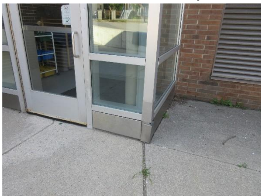
Alum. Curtain Walls & Doors- Minor damages & gaps between pressure caps
