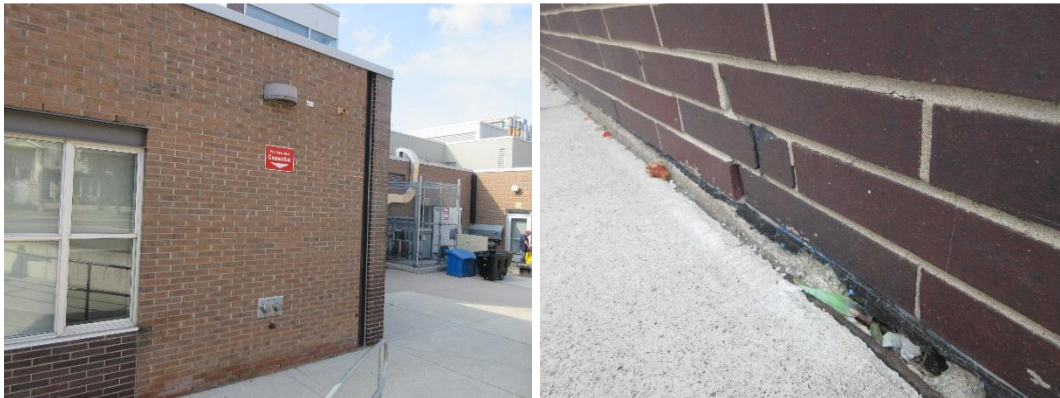
Brick conditions- deterioration/ damage at grade
