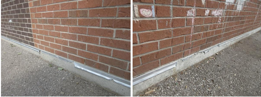
Damaged flashing at grade
