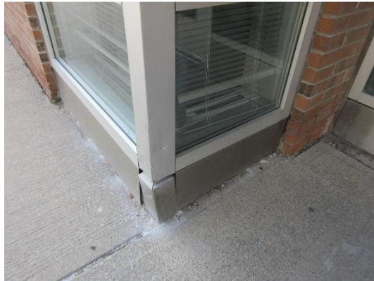
Damage and gaps have developed in a number of locations throughout curtain wall areas
