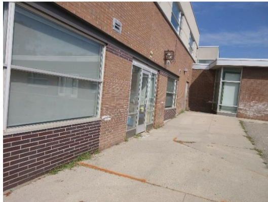
Staining/rust at grade- Aluminum doors & steel columns
