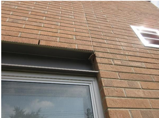
Exposed steel columns & Beams as window surrounds
